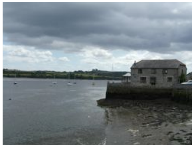
This quay storehouse (now a private dwelling named The
